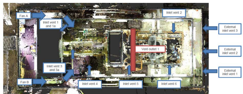
Kings Lynn Ventilation ducting layout shown for GT enclosure, fans and air intake/ouptake
