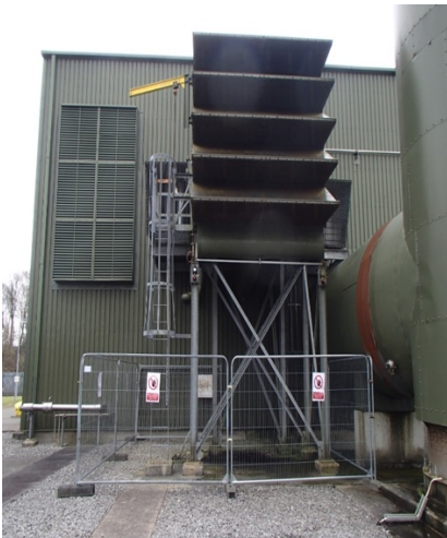
Safety cordon to prevent injury risk from corrosion of the intake
